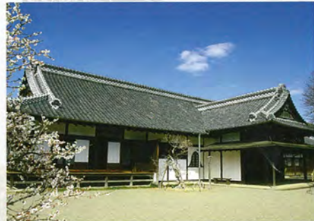
Kodokan (Kodokan school/1841-1872/ Mito City, Ibaraki Prefecture)
